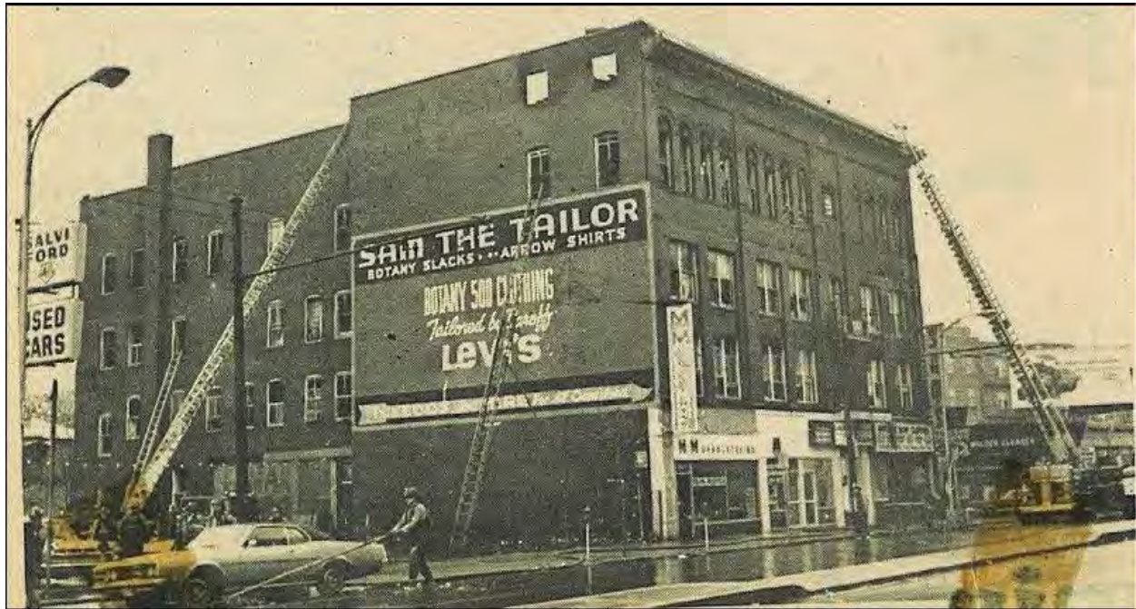
I.O.O.F. Building formerly located at 2072 Massachusetts Avenue, depicted during the 1968 fire which led to its demolition ( Cambridge Chronicle ).
