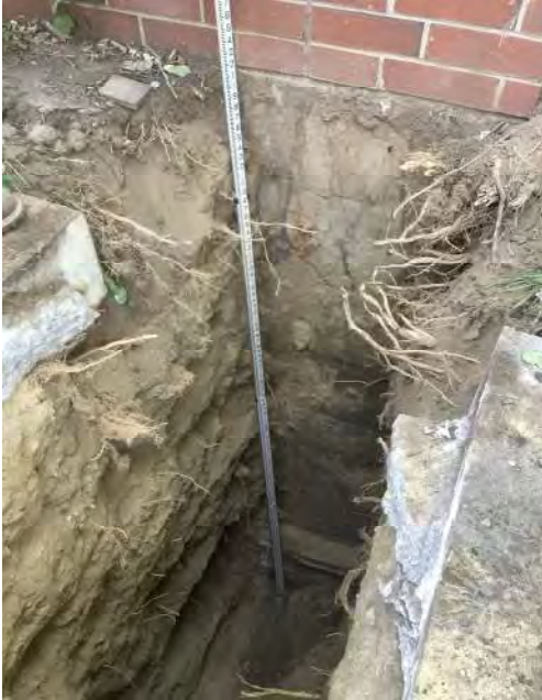
Photograph No. 1: View facing 2050 Mass Ave foundation wall.
