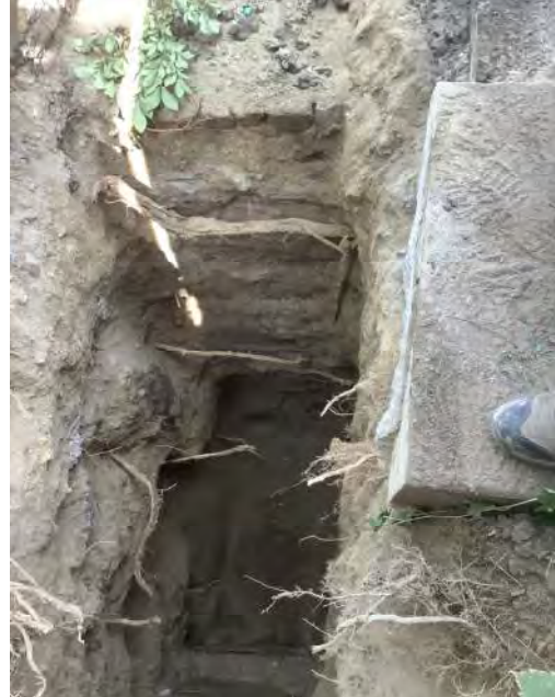
Photograph No. 2: View facing existing foundation wall in site (2072 Mass Ave).
