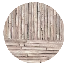
MASONRY SOLDIER COURSE AT HEADER
