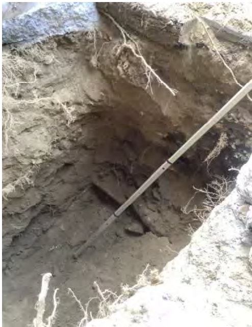
Photograph No. 5: View facing brick foundation wall in site (2072 Mass Ave).
