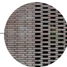
OPENINGS IN MASONRY FACADE
