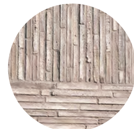
MASONRY SOLDIER COURSE AT HEADER
