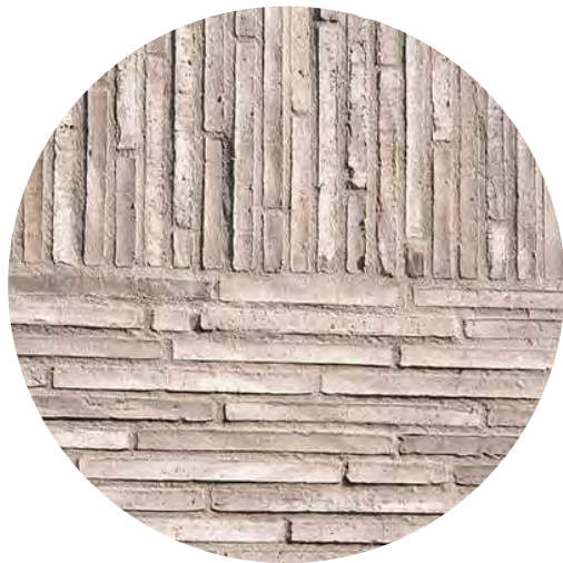
CONTEMPORARY INTERPRETATION OF BRICK AT "LINTEL"
