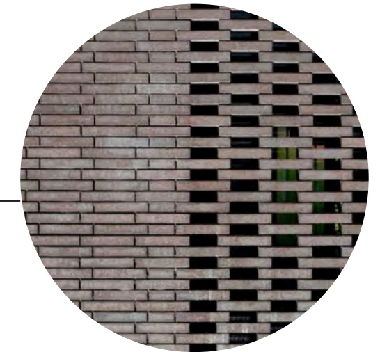
OPENINGS IN BRICK FACADE
